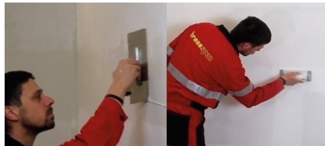
Picture No. 9: Covering of the edges.
