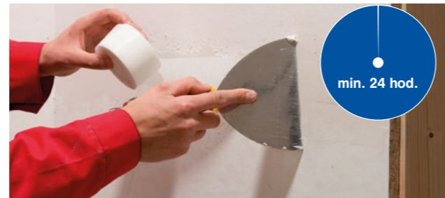
Picture No. 8: Covering of the edges.
