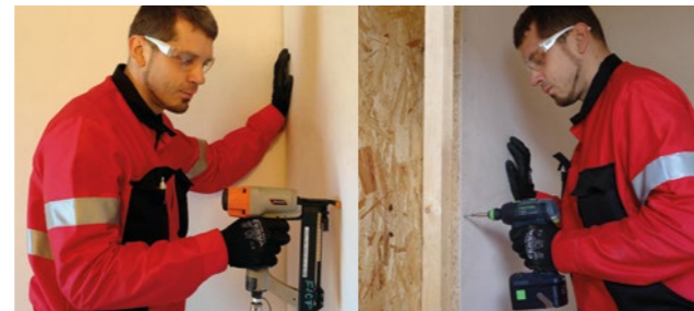
Picture No. 6: Nailing, stapling.
